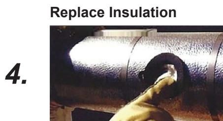
Insert insulation into hole. Flexible insulation is recommended such as fiberglass or mineral fiber.
