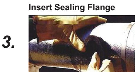
Insert the sealing flange portion of the inspection port into the pre-cut hole in the insulation cladding. On smooth metal the cladding should fit between the outer lip and the first locking undercut. For corrugated applications it should be held into position with the lower locking undercut.
